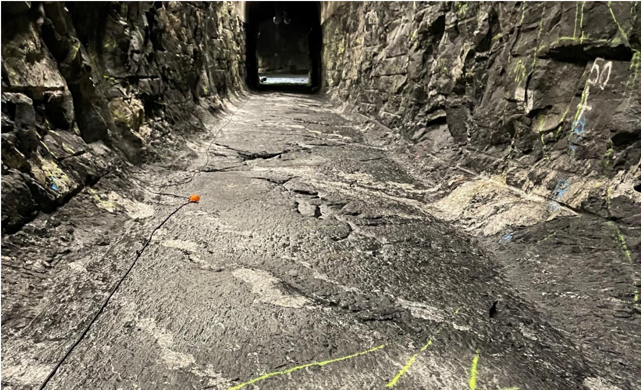
Figure 4-1. A deposition tunnel in ONKALO, picture Timo Saanio.
